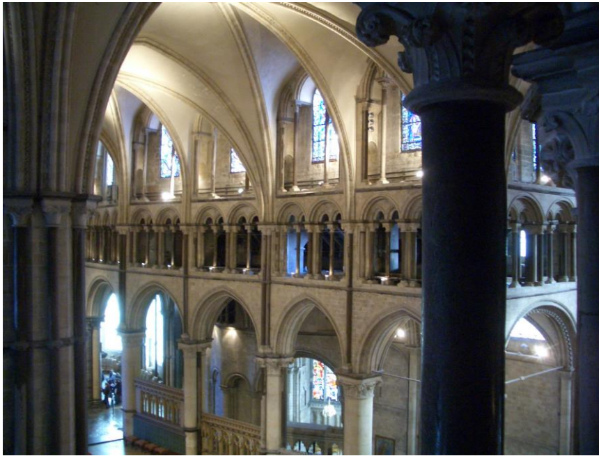
FIGURE 2: THE LATE 12TH CENTURY TRIFORIUM GALLERY (CENTRE) AND CLERESTORY WALL-PASSAGE (TOP) IN THE CHOIR OF CANTERBURY CATHEDRAL
