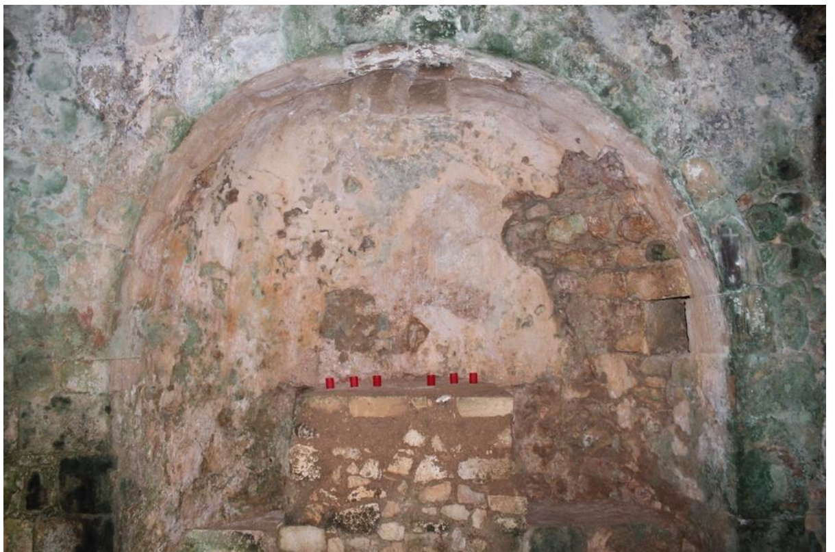
Fig. 17. Cylindrical apse made of ashlars and wet rubble containing a stone altar, Cave church of St. Leonard.
