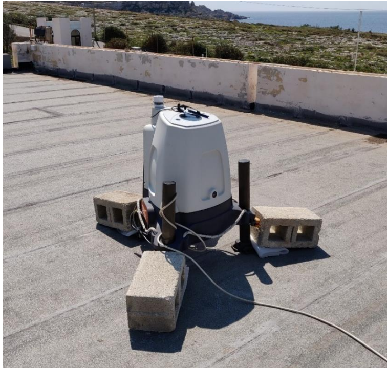
Figure 4.14: The ZephIR 300 LiDAR unit installed on the rooftop of the WSC-RO Plant, at Ċirkewwa, l/o Mellieħa, Malta.
