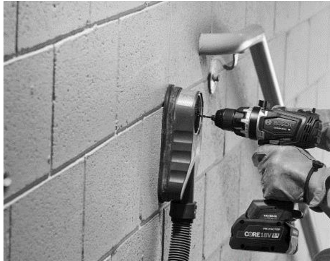
Figure 1: Drilling a hole in a brick wall using a cordless drill (Source: https://www.facilitiesnet.com/ )
