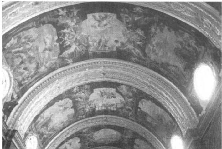
Fig.2 - St. John's Co-Cathedral, Valletta. Section of the vault, painted by Mattia Preti
