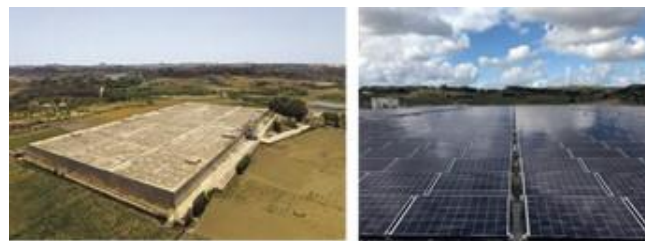
Figure 2: Good-practice example of solar photovoltaic communal farm in Malta.
